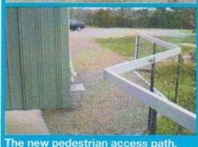
The new pedestrian access path.
